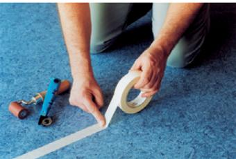
Clean the seam area and fix a **special**, even masking tape, which is resistant against our cold-welding liquid, centred over the closely cut seam. This is absolutely necessary to avoid damage to the floor finish (e.g. made of Polyurethane) of the floor covering.
