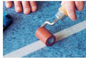
Easily cut the masking tape with the rolling knife in the seam area. Alternatively a straight blade or a hook-blade can be used. It is important not to damage the edges of the floor layers while cutting the tape. This can be done effectively by pressing the knife deeply into the seam, resulting in a good guidance.
