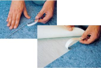
After the double cut remove the cut-offs of the upper and lower layer.
