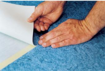
In case the PVC-floor covering is not glued holohedral on the floor (please consider the manufacturers recommendations), the seam area has to be fixed to the surface by using a proper double-sided adhesive tape. Press the floor layers, which have to be laid tightly, firmly onto the double-sided adhesive tape.
