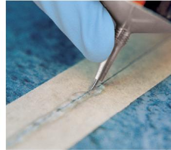
After about 10 minutes the cold-welding liquid on the masking tape is dry and the tape has to be removed steadily backwards at an angle. Swellings in the seam area of the PVC-floor covering will decrease. The result is a barely perceivable seam with a high seam tensile strength. The seam can be walked on after about 30 minutes.
