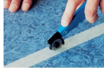
In case of hard and little flexible PVC-floor coverings (for instance Commercial Floor Coverings) warming up the seam area (to a maximum of 40°C by using a blow dryer or an iron) before welding enables an easier and more even guidance of the needle in the seam.
