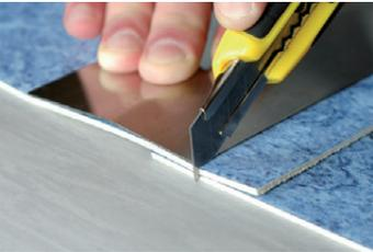
The overlapping laid floor layers (3 to 5 cm) will be cut in one step alongside a metal bar (double cut).
