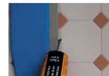
PVC-Wallpapers can be welded by using the aluminium nozzle which is included. Remove the plastic stopper; it is meant for cleaning the nozzle. Bring the aluminium nozzle evenly and centred onto the seam and apply the PVC-cold-welding paste steadily, working from top to bottom alongside a straightedge. The volume of the applied paste reduces about 75 % while drying, therefore do not wipe off any paste but let it dry (about 30 minutes).
